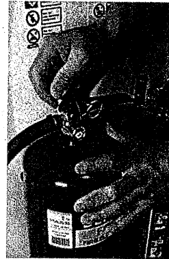
One indicator the fire extinguisher is charged and serviceable is the pressure gauge needle will be located in the green.
